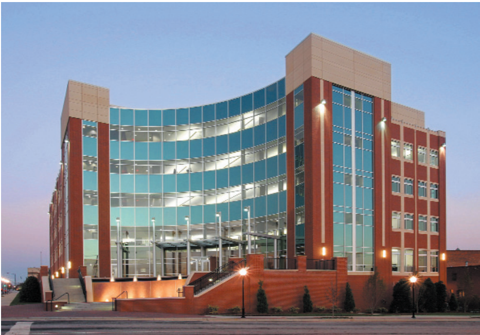
In commercial buildings, the ideal energy-conserving glass would let in the majority of the visible portion of the solar energy-- thus allowing reduced lighting requirements in the building, while blocking most or all of the UV radiation and infrared night.
